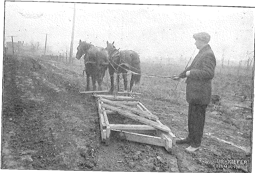
FIG. 9. — Method of hitching to drag in moving the same to or from where it is to be used on the road.
