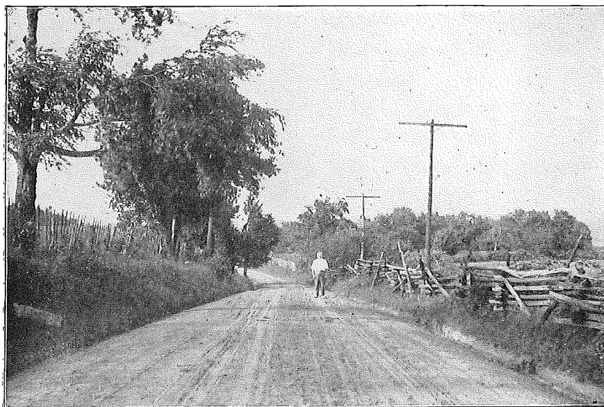
FIG. 14. — A well maintained earth road. The above results are secured by proper drainage and by dragging with a cheap road drag.
